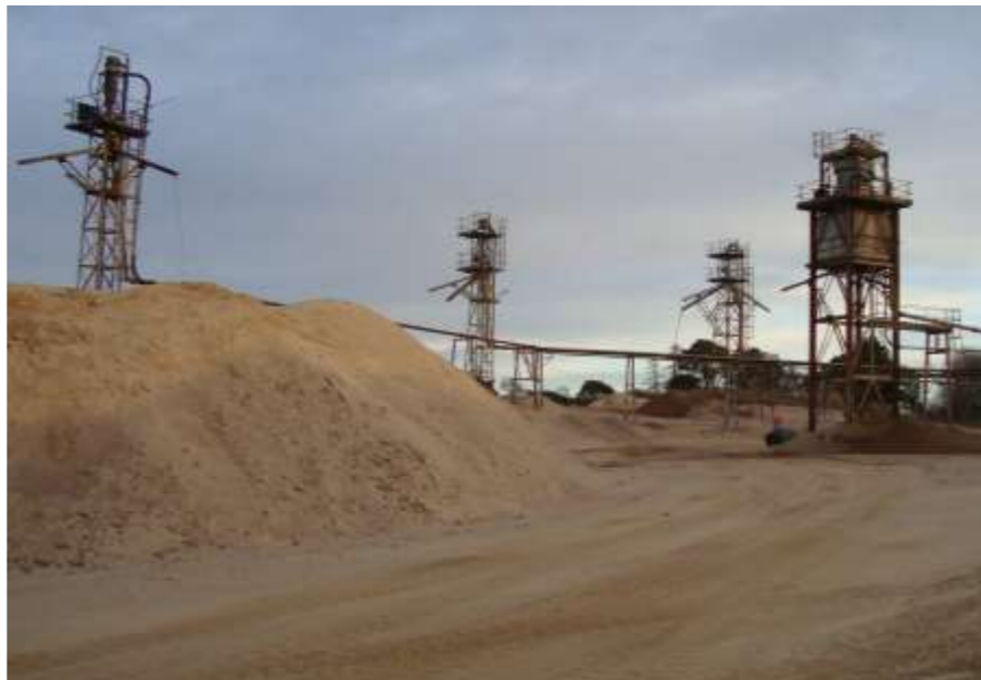
Small scale industrial structures within Park Quarry
