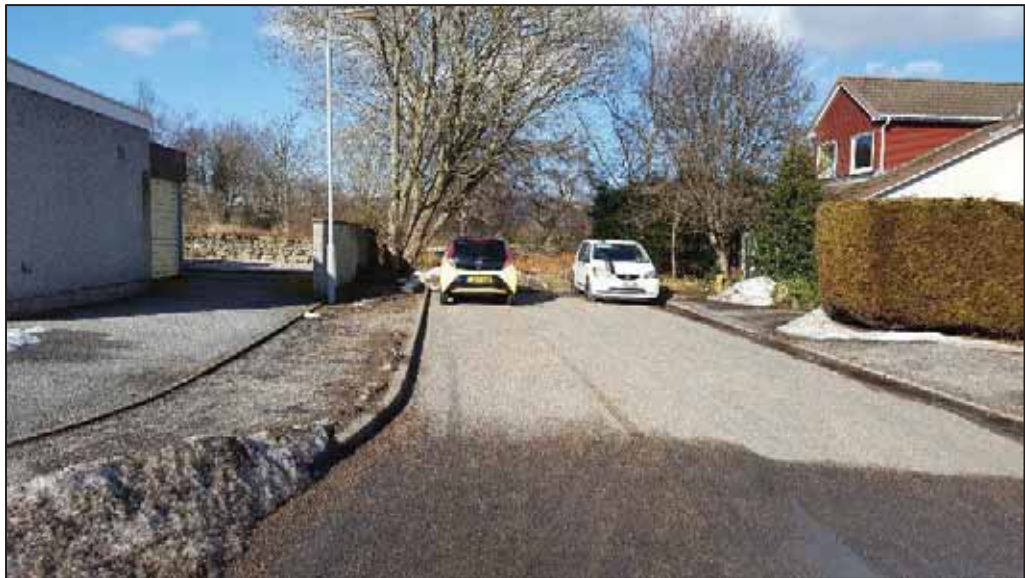
Footways on Hillview Road
