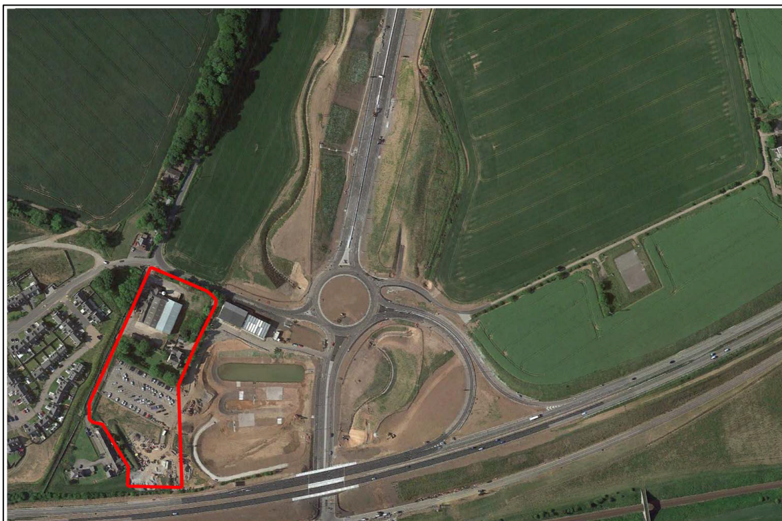
Figure 4 – Aerial Photograph of Site KN115
