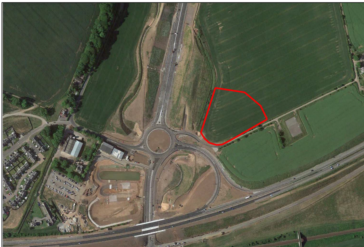
Figure 8 – Aerial Photograph of Site KN119
