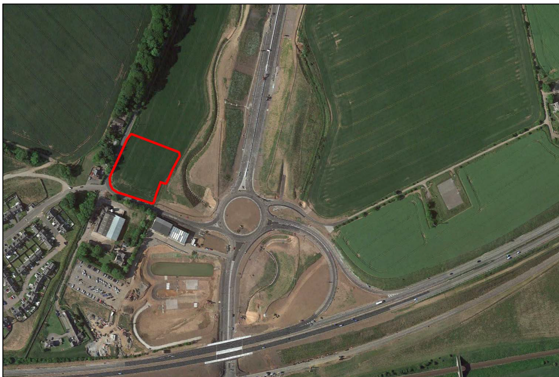
Figure 6 – Aerial Photograph of Site KN118
