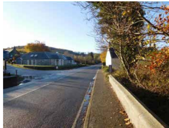
Figure 8b: B9077 at bridge crossing
