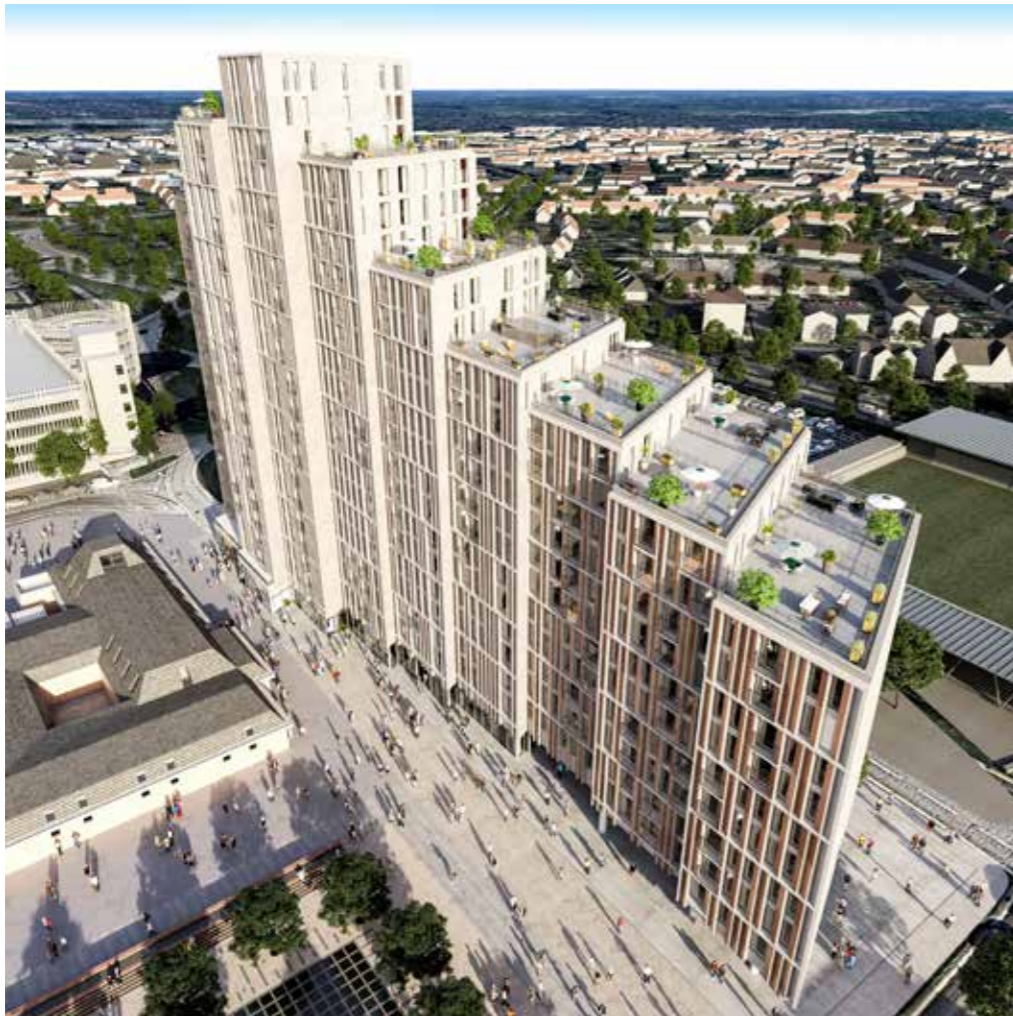
Royal Winchester House, Bracknell Residential Masterplan Project Stage: Construction
