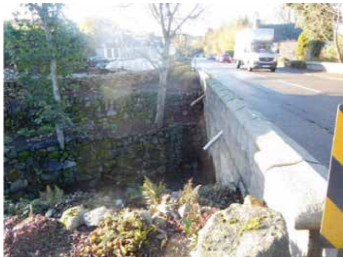
Figure 8a: B9077 bridge crossing
