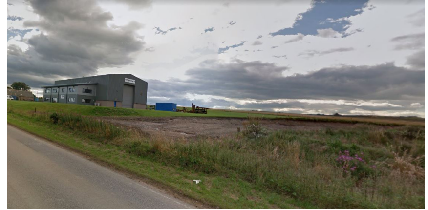
1 — View looking South West over proposed site B by Rashierieve Foveran
