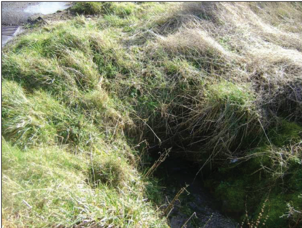
Photograph 20: Ditch D inflow culvert under Stonehaven coastal road (assumed 0.25m dia. pipe culvert).
