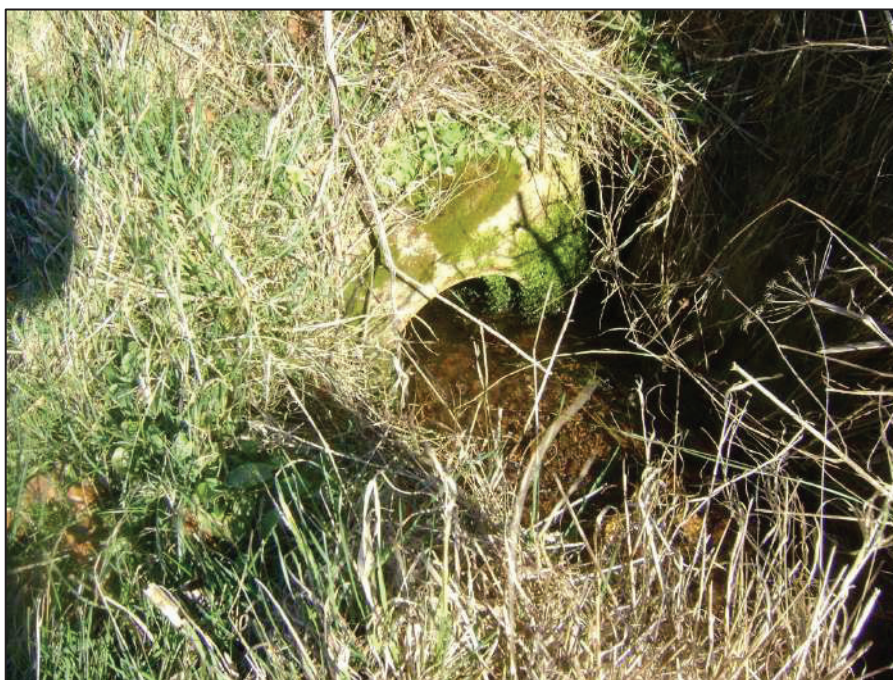
Photograph 2: Ditch A inflow culvert under A92 (300mm dia. clay pipe)
