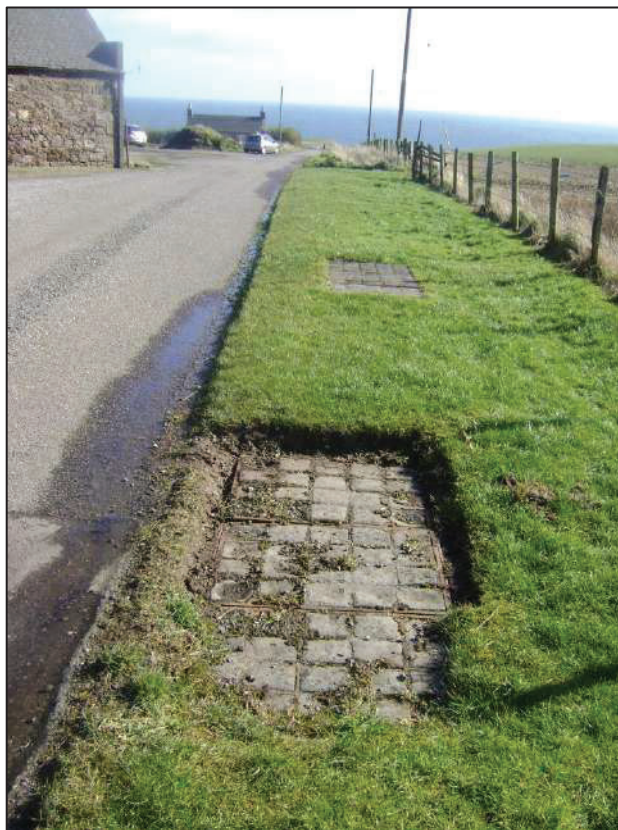
Photograph 18: Looking downstream along culverted section of Ditch D at farm (assumed 250mm clay pipe culvert)
