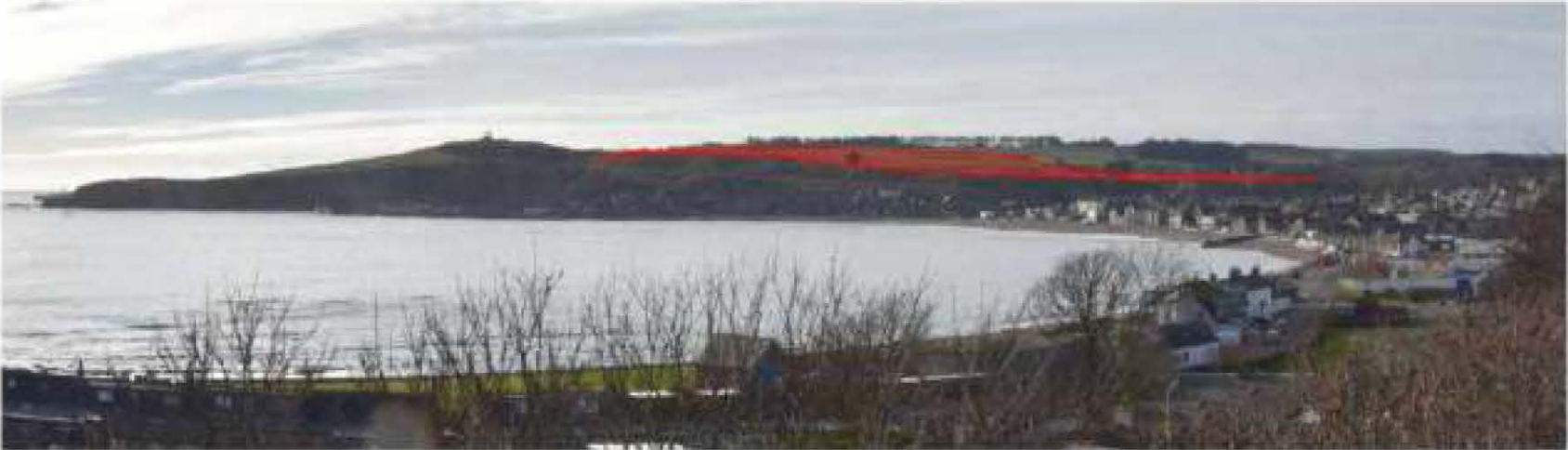
LOOKING SOUTH FROM LAY-BY OF BRAESIDE CRESCENT
