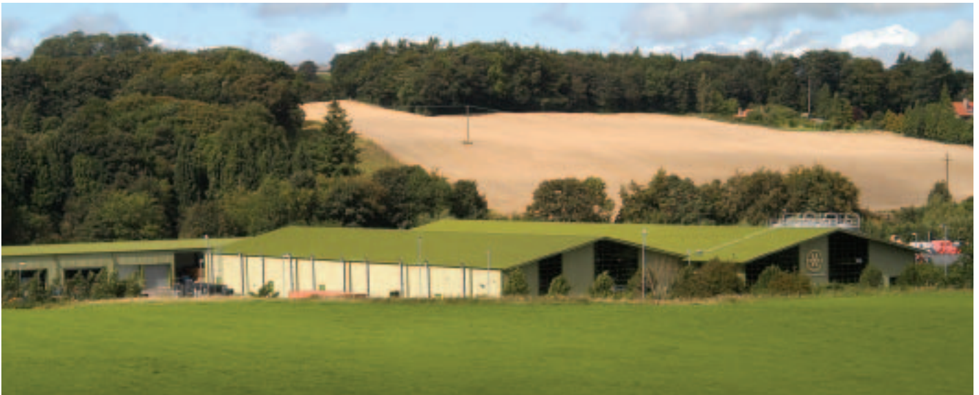
Emtelle UK Ltd, Fibre-optic Research Centre, Hawick
