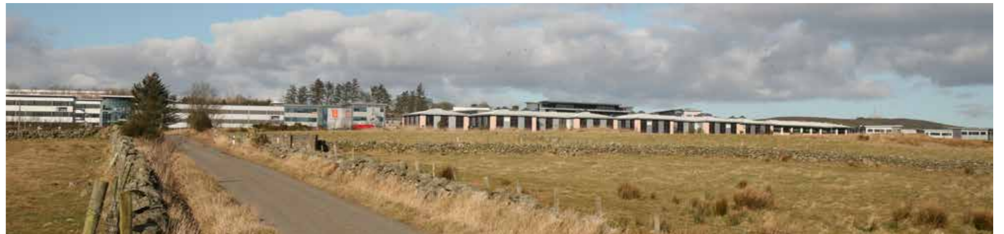
Large floor-plate buildings with significant visual impact
