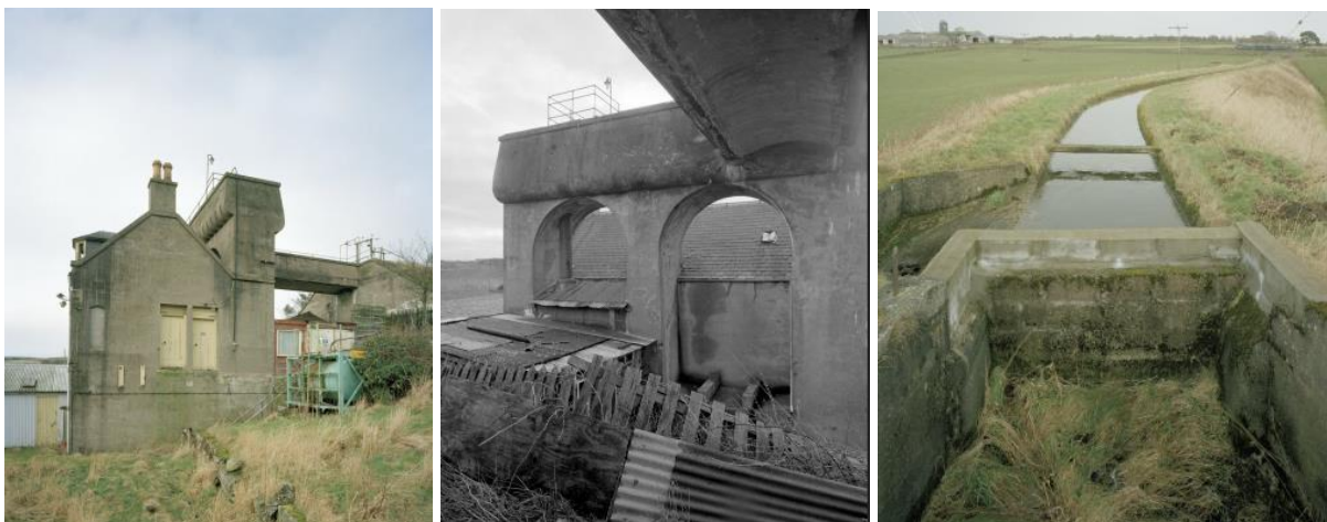
Figure 8 – Parkhill Pumping Station
