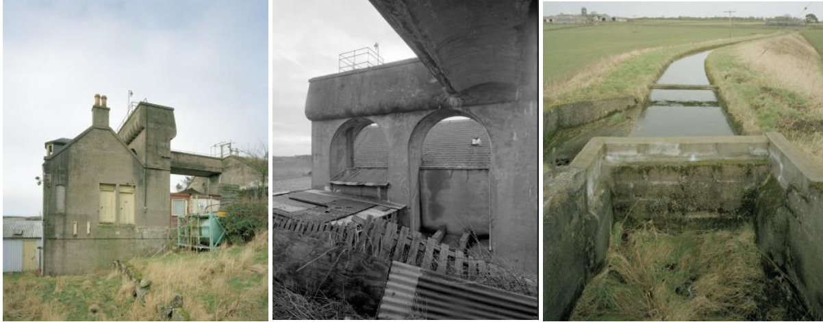
Figure 8 – Parkhill Pumping Station
