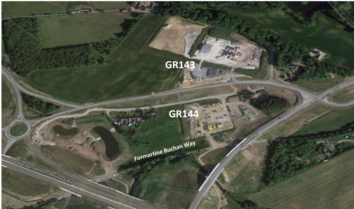
Figure 6 – Further Site Aerial (Source: Google Maps) showing relationship between sites and the new road network, including access to the Formartine Buchan Way cycle route.
