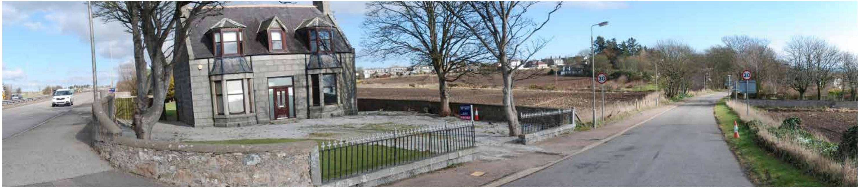
3 View looking north east from the junction of Walker Drive and the A92.
