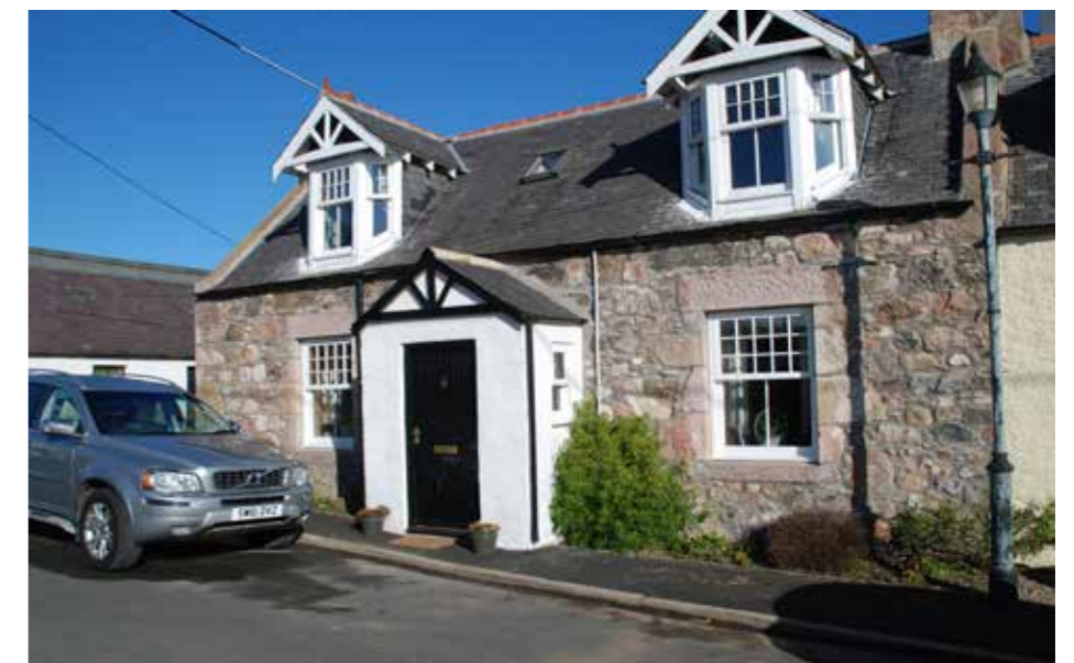
1.5 storey terraced cottage with exposed stone facade
