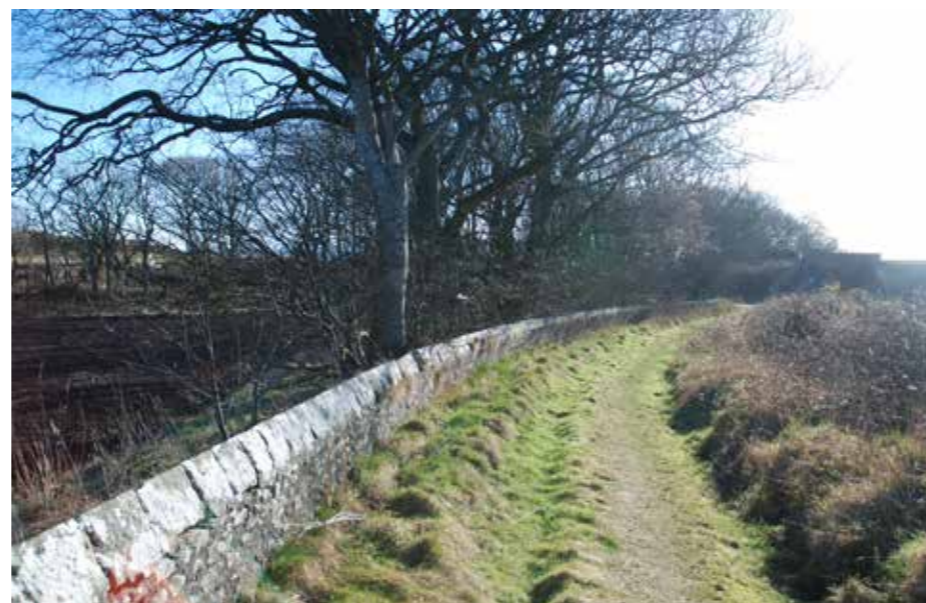
Stone walls with distinct pointed coping at the edge of the village
