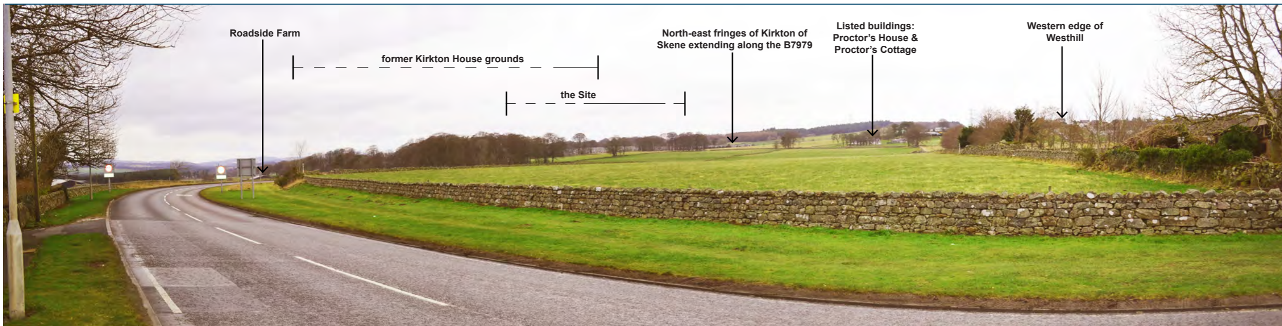
VIEWPOINT 1: Middle distant view looking north-east towards the Site from the A944, Straik Road, on the western edge of the small village of Mason Lodge. Intervening mature landscape features including policy woodlands across the former Kirkton House Estate and Easter Skene Estate, tree belts defining field boundaries and the ancient belt of trees creating an avenue effect along the Old Skene Road combine to contain views towards the western sector of the site and filters views towards the eastern sector. Where visible any new housing would be seen in the context of the existing built edge of Kirkton of Skene and would not exceed the visual urban envelope of the village from this location.
