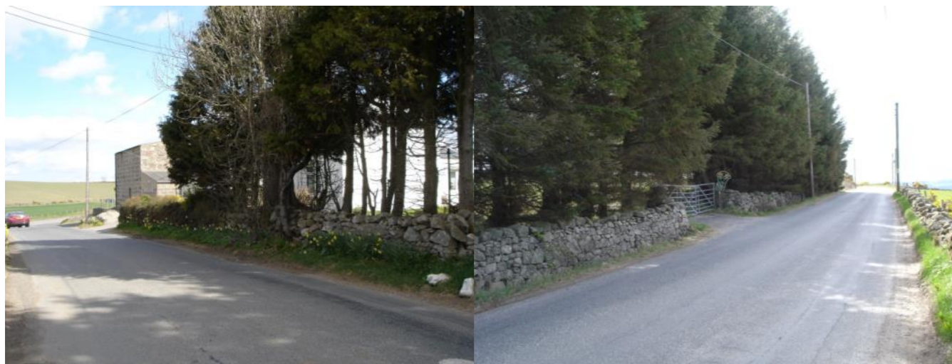
3. View to edge of the site from Hill of Keir Road— existing access and boundary planting
